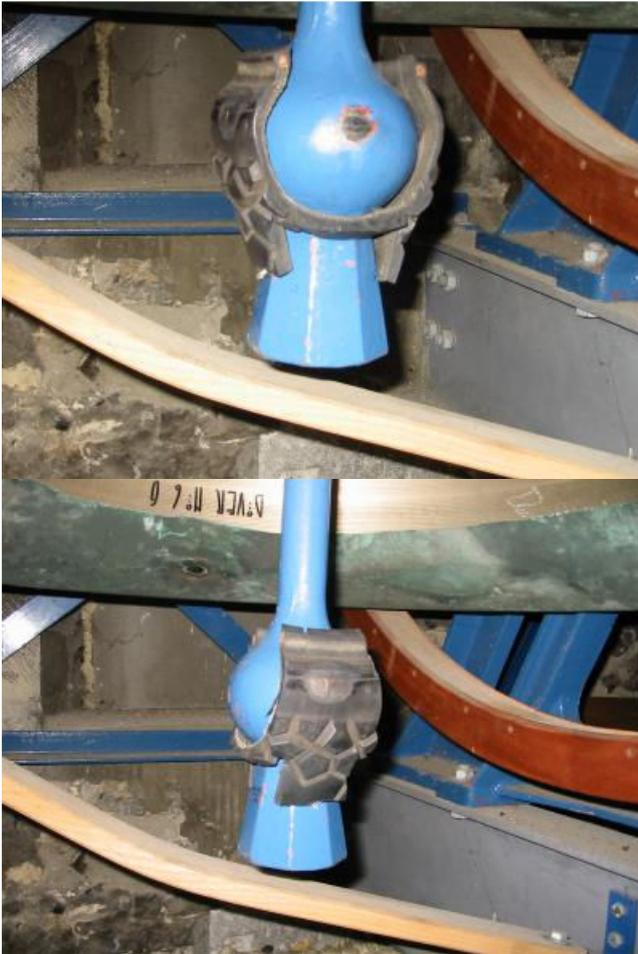
With the tyre as shown in fig 7a, the clapper strikes the bell normally.
